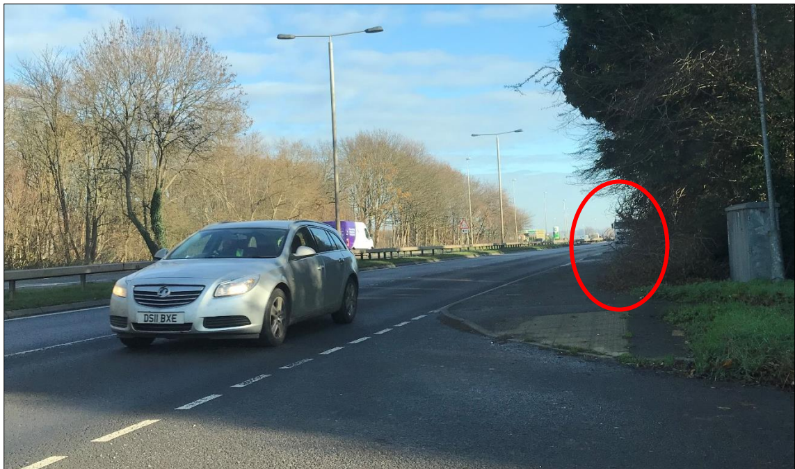
Image 4 – Overgrown Vegetation at the Bassingfield Lane Junction
